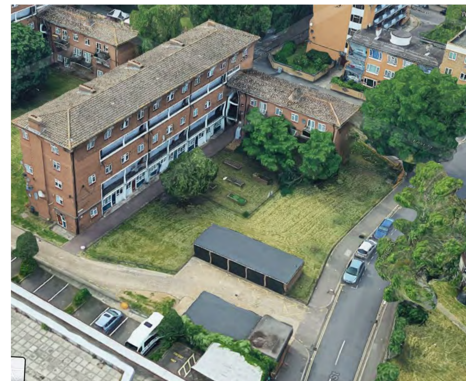
AERIAL VIEW OF EXISTING SITE - FROM SOUTHEAST
